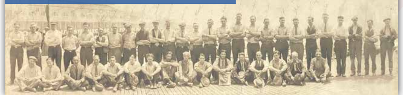
Local 5 members working for Otis Elevator Company on construction of the Haddon Hall hotel (now Resorts Casino) in Atlantic City in 1929, the year it was completed.
